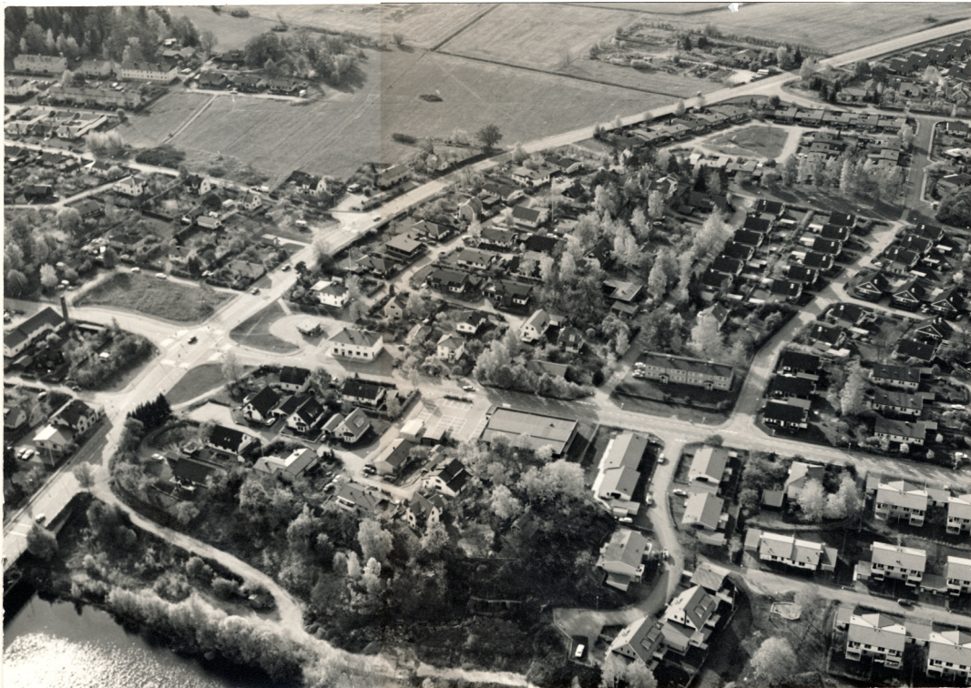
Hjulsbro centrum. ① Hjulsbro EL. ICA-Flamman.DIN-Kiosk.
